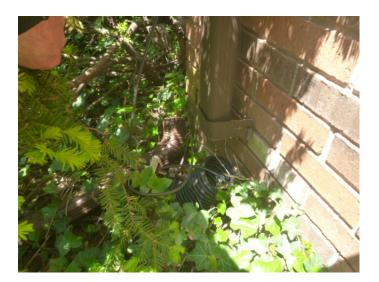
Gutters and downspouts are an integral part of a homes storm water management system and should be monitored on a regular basis for proper operation. It is recommended that the gutters and downspouts be cleaned and flushed as part of routine maintenance to reduce the potential for water backup and resultant damage to roofing materials and concealed portions of the home.
