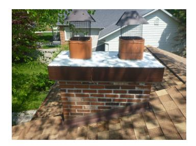
Step# **Comment** Component 1401. Chimney Type Masonry chimney. 1402. Visible Suggest sealing chimney cap (chimney crown) to reduce Condition opportunity for water infiltration and damage. This is a common maintenance item that is often neglected by homeowners; you should make a crown inspection part of your routine seasonal maintenance checklist. 1403. Chimney Flue Clay. 1404. Flashings
